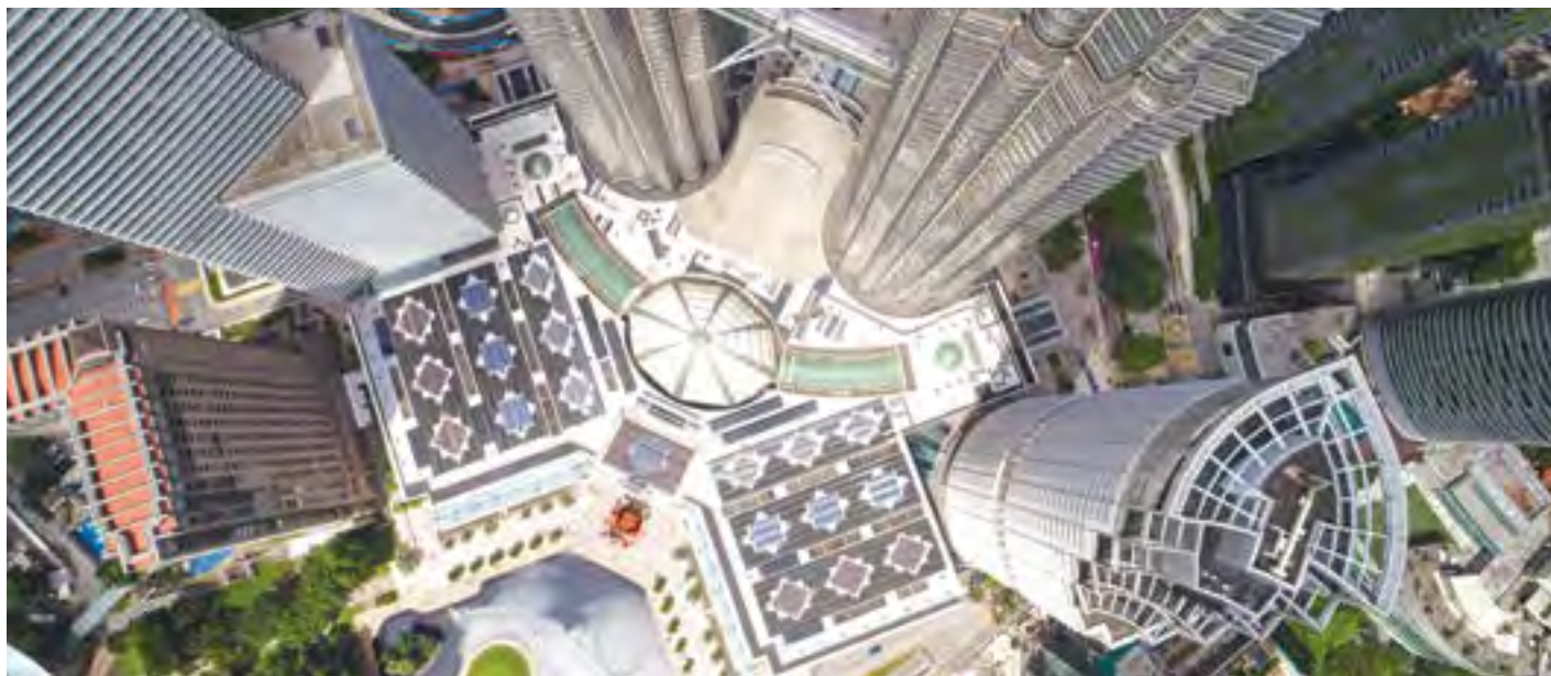
↑ Solar Photovoltaic panels on the rooftop of Suria KLCC
