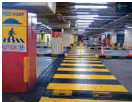
Speed humps and pedestrian crossings are placed at strategic locations within the KLCC's North-West Development car park for customers' safety.
