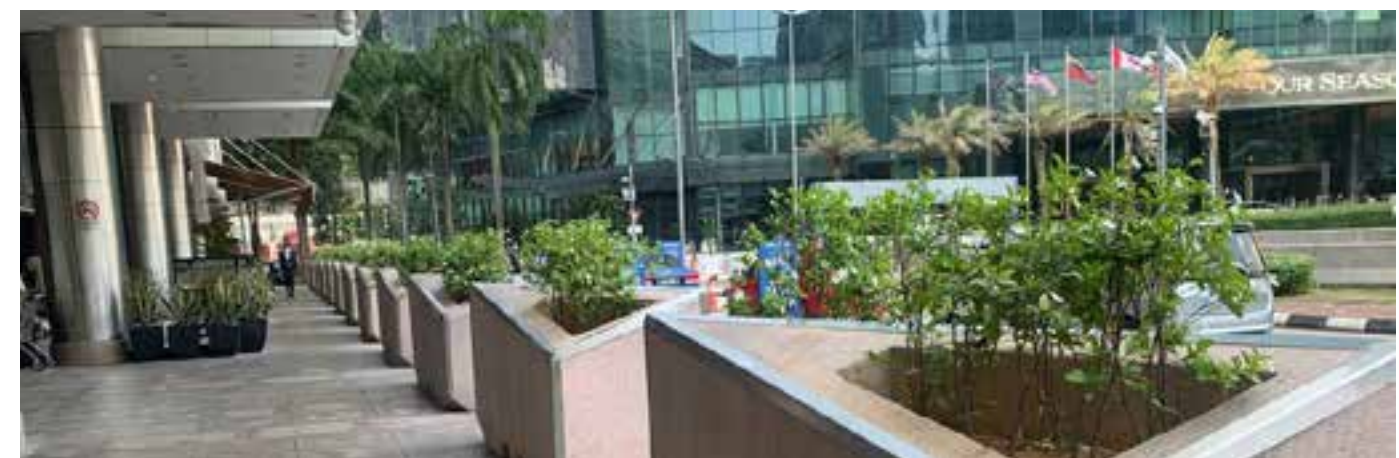
Planter boxes installed at Suria KLCC to provide Hostile Vehicle Mitigation.
